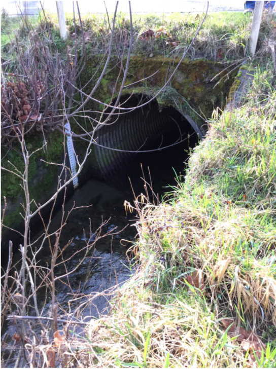
Graphic 2. Existing Culvert Outfall (48" CMP)
