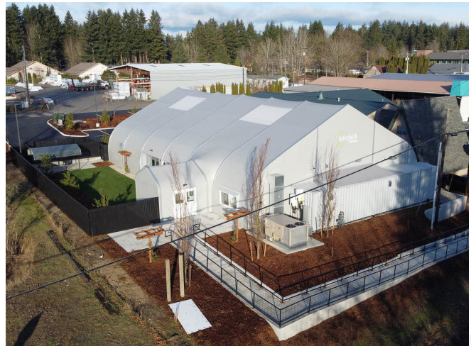
Sprung Shelter, Washington
