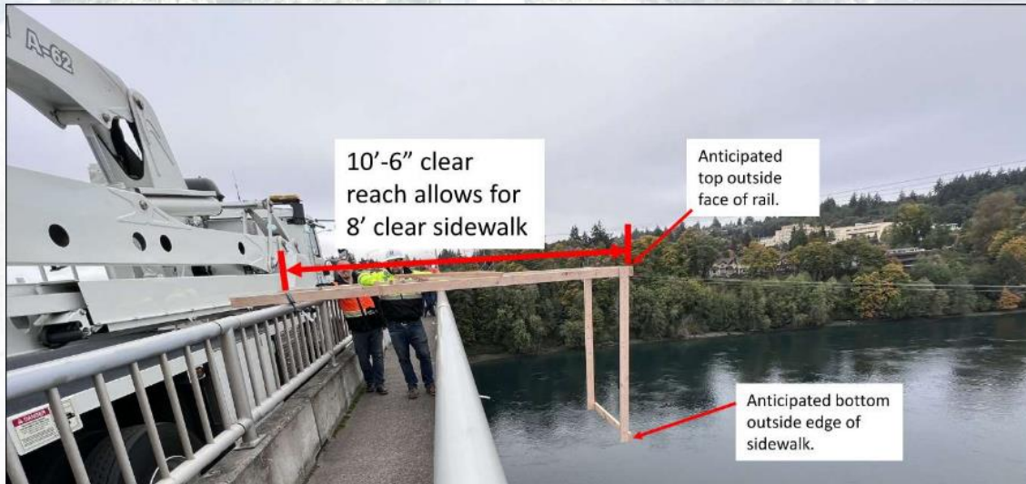
WSDOT Field Test – Looking North
