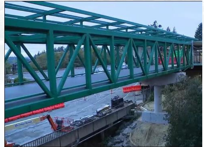
New FRP Decking at Bainbridge Ferry Terminal
