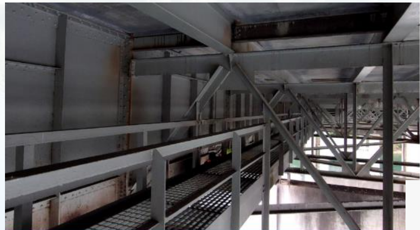
Existing catwalks on the Warren Ave Bridge
