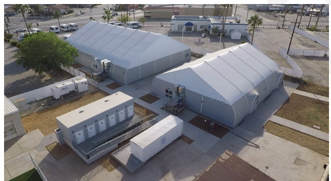
Sprung Shelter, California
