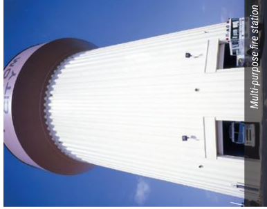
Dual storage - 620,000 gallons upper tank and 1,130,000 gallons lower tank. (SIT/SPA Tank of the Year)
