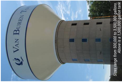
Concrete support structure requires minimum maintenance on both inside and exterior
