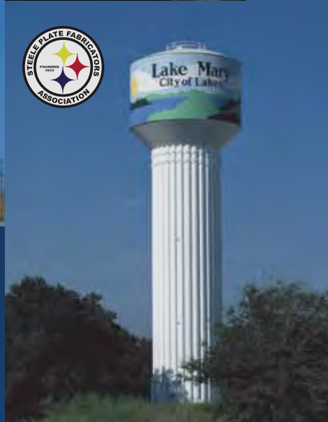
500,000 Gallon Lake Mary, Florida Steel Tank of the Year 2002 - Steel Plate Fabricators Association
