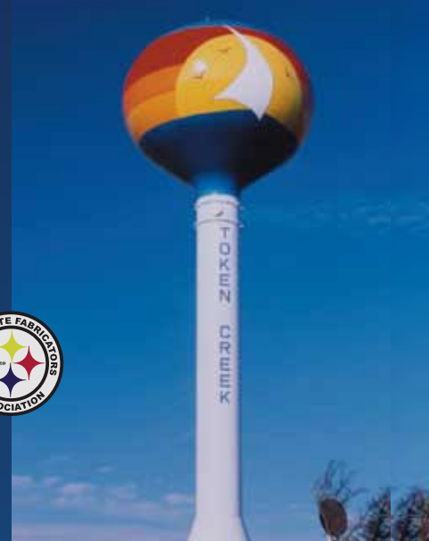
200,000 Gallon Burke, Wisconsin Steel Tank of the Year 1995 - Steel Plate Fabricators Association
