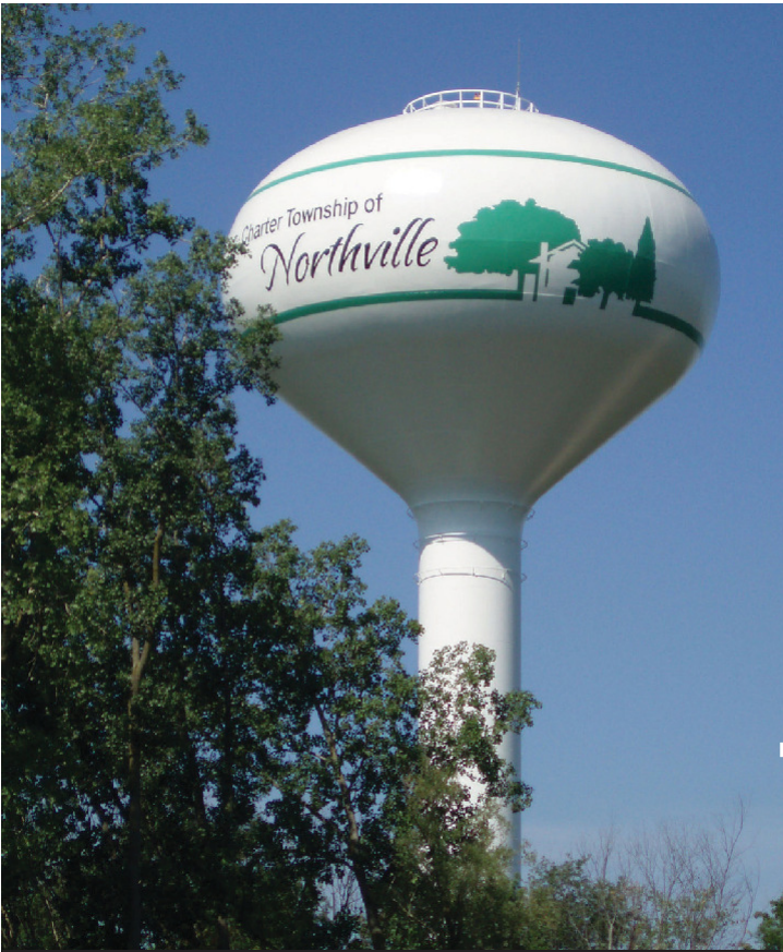
Northville, MI – 1,000,000 gallons
