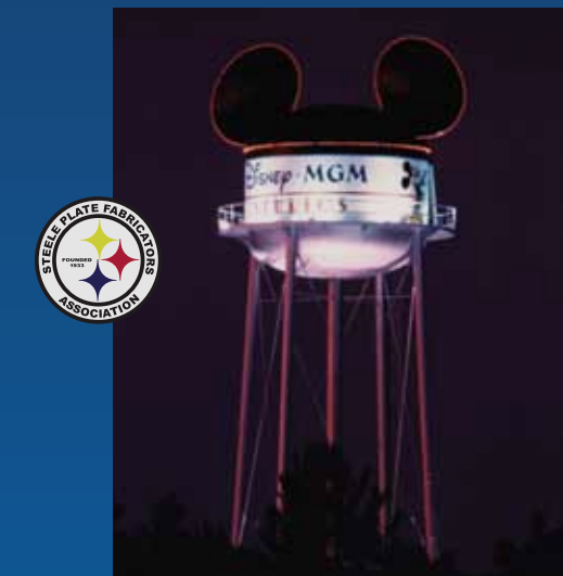
150,000 Gallon Double Ellipsoidal Lake Buena Vista, Florida Steel Tank of the Year 1987 - Steel Plate Fabricators Association
