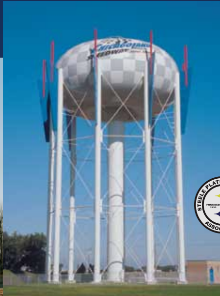
1,000,000 Gallon Torus Bottom Joliet, Illinois Steel Tank of the Year 2001 - Steel Plate Fabricators Association
