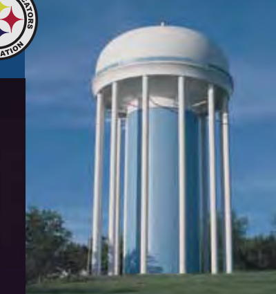
1,500,000 Gallon Antebellum Newnan, Georgia Steel Tank of the Year 1998 - Steel Plate Fabricators Association
