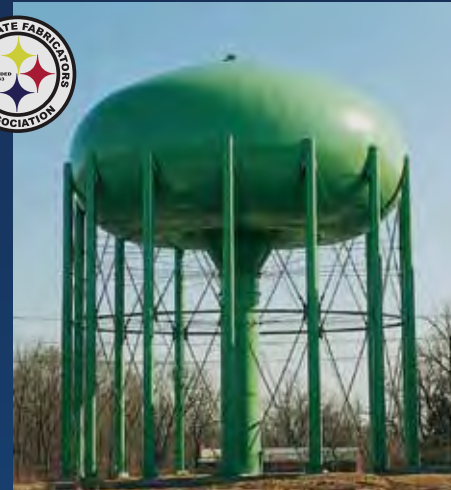
2,000,000 Gallon Torus Bottom Montgomery County, Ohio Steel Tank of the Year 1993 - Steel Plate Fabricators Association
