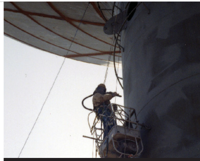
Unhindered maintenance access
