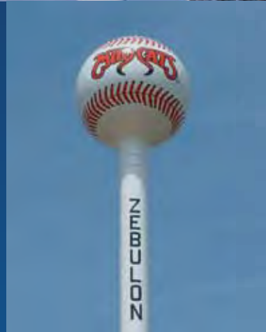
200,000 Gallon Zebulon, North Carolina
