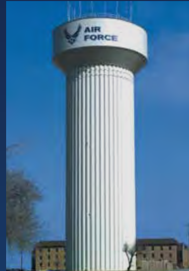
1,000,000 Gallon McConnell AFB, Wichita, Kansas
