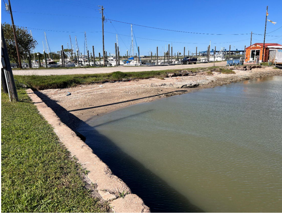
Looking North from Seawall at location of proposed future fishing/crabbing dock and transient boat slips. Photo taken 10.15.2023
