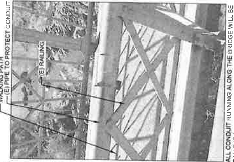
ALL CONDUIT RUNNING ALONG THE BRIDGE WILL BE RUN THROUGH EXISTING PIPING THAT IS ATTACHED TO THE RAILING AT THE PEDESTRIAN PATHWAY
