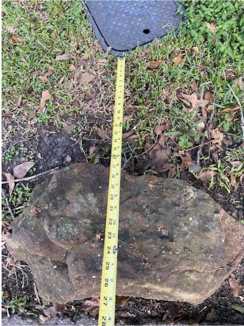
City box for water line flush valve is 27 inches from the street
