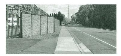
Figure 1: Existing 8 ft. concrete paneling fencing along E. Front Street at Lynden Substation
