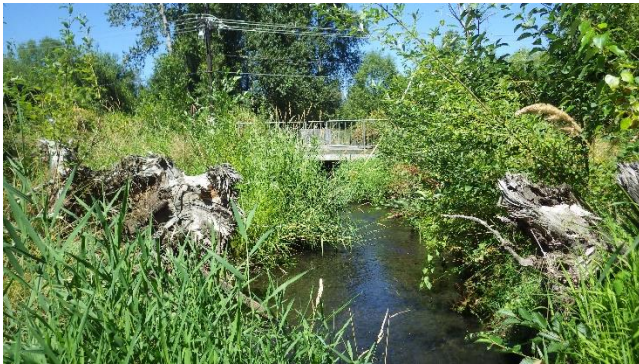
Integrated stormwater and pathway create a park-like atmosphere.
