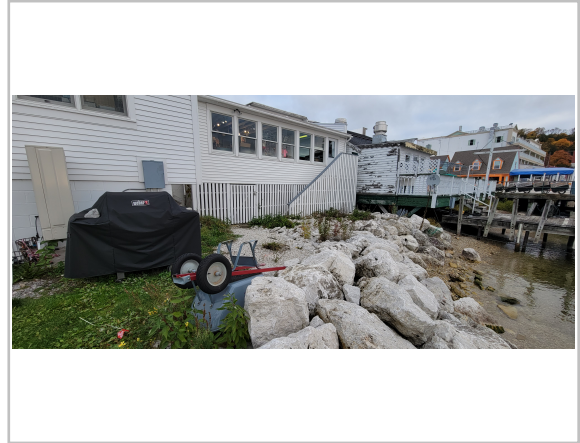
Photo: 14 Looking: N Taken: 10/22/23
