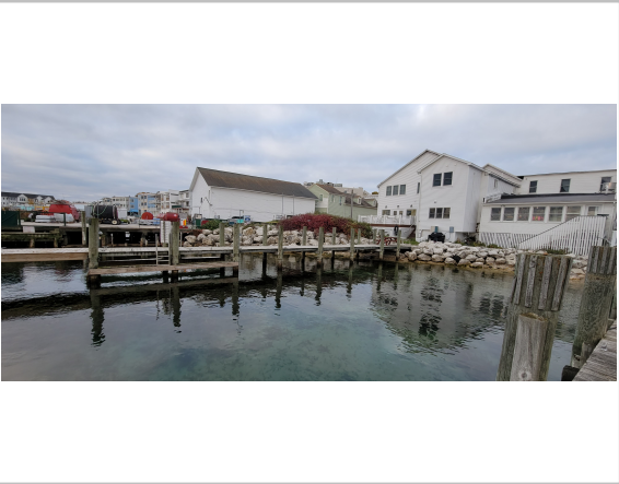
Photo: 13 Looking: W Taken: 10/22/23
