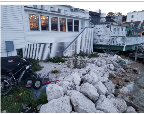
Photo: 17 Looking: N Taken: 10/13/23
