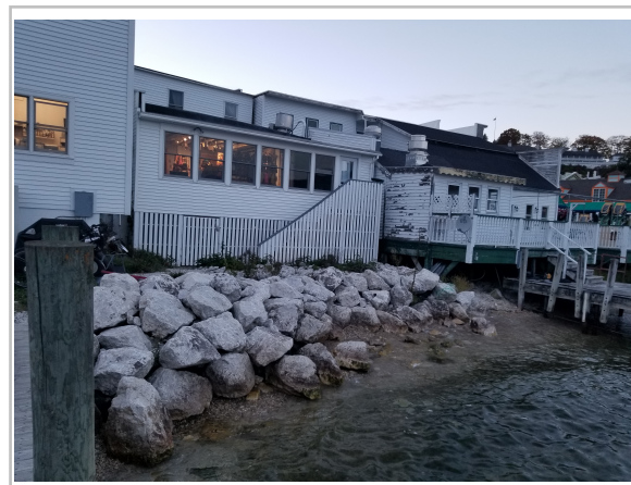
Photo: 18 Looking: N Taken: 10/13/23
