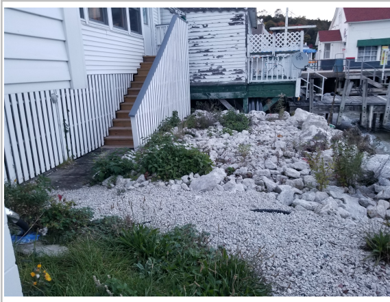
Photo: 19 Looking: N Taken: 10/13/23
