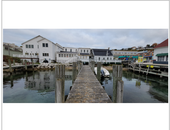
Photo: 10 Looking: W Taken: 10/22/23
