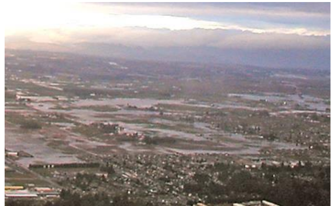
North Lynden Flooding (looking north)
