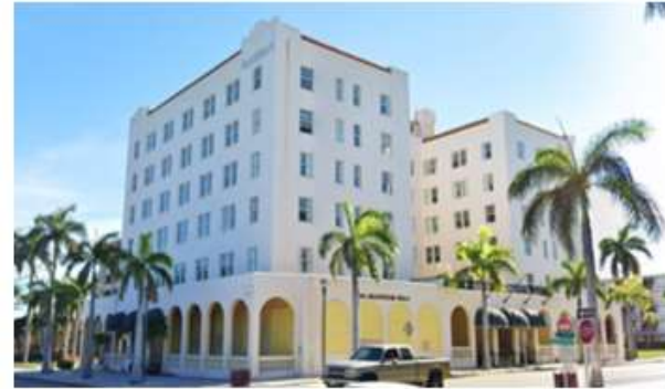
Gulfstream Historic Hotel. Google Maps Street View
