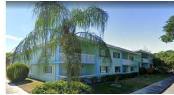
499 Lakeside Drive. Google Maps Street View
