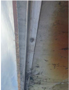
All "A" grate structures, A3, Midfield and A5 on Alpha Taxiway side have 2"x2" aluminum angle supported with bolts on the structure.
