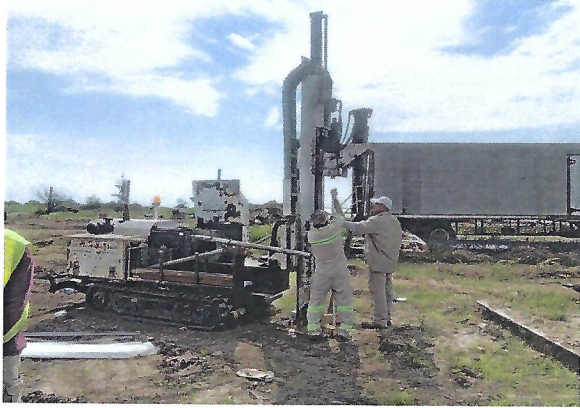
No. 5 View of SB-3 location at the north central portion of the site.
