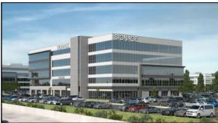
LASALLE BUILDING (under constr)
