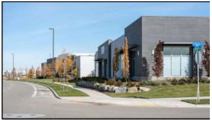
EXISTING SINGLE-STORY SHOPS
