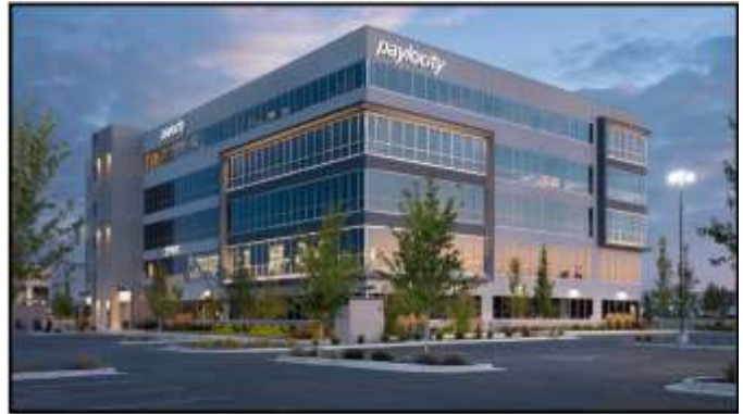
PAYLOCITY BUILDING (complete)
