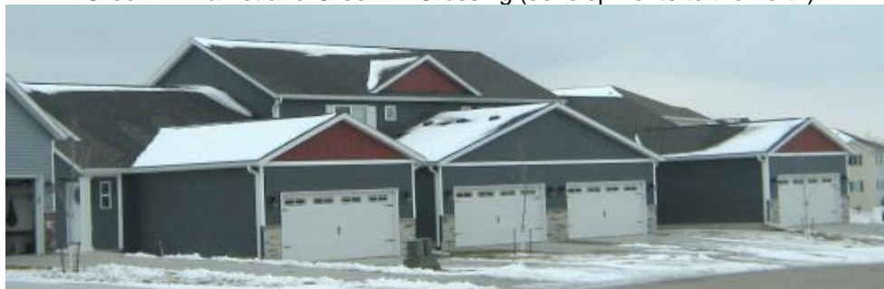
Greenhill Village Commercial 4th (development to the east)
