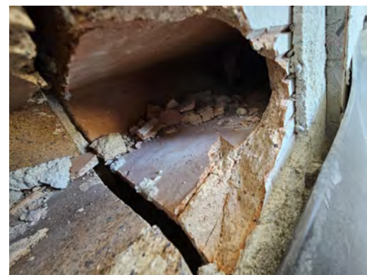
No reinforcement in clay/masonry walls
