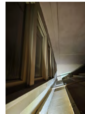
Hidden clerestory windows lack of shear transfer between roof diaphragm and shear walls below
