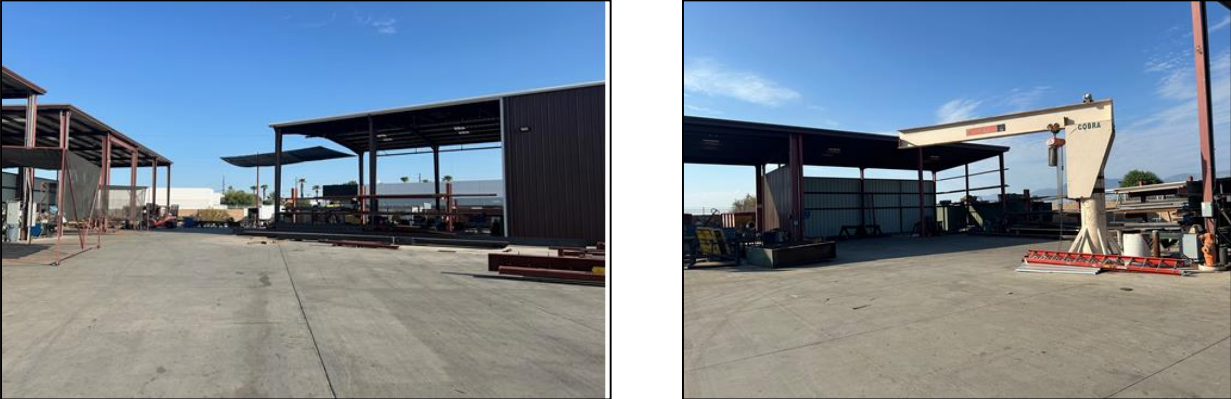
Figure 1 and 2: Photos of Site Metal Canopies
