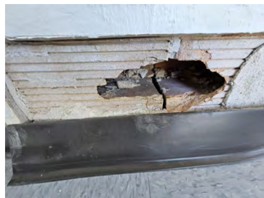
No reinforcement in clay/masonry walls
