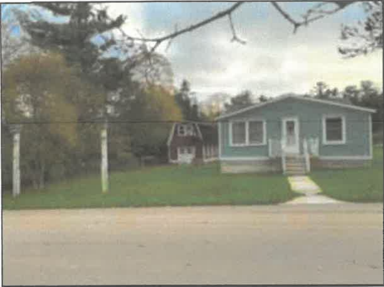
Existing House East
