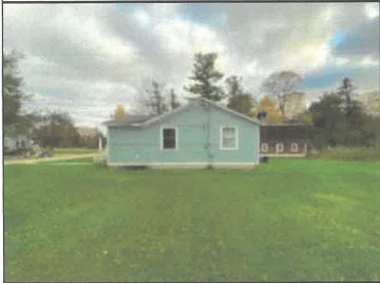
Existing House North
