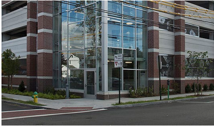
Using Articulation and Landscaping of Non-Programmable First Floor. SOURCE: Top-MTA of the State of New York; Bottom-Nyttend
