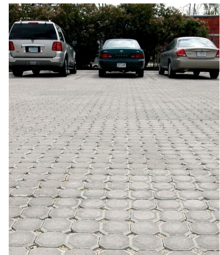
Pervious Paving. SOURCE: Jason Johnson
