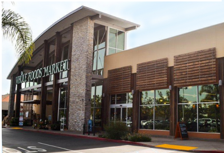
Frequent Changes in Façade. SOURCE: Michael Baker International
