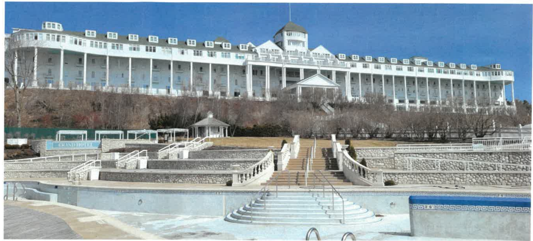
EXISTING SOUTH FACADE OF HOTEL
