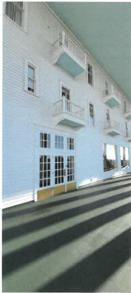
EXISTING VIEW PORCH FACADE
