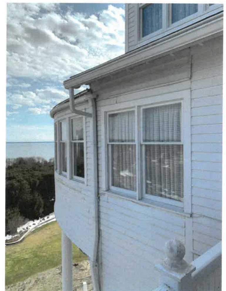
EXISTING VIEW OF EAST END 300 LEVEL
