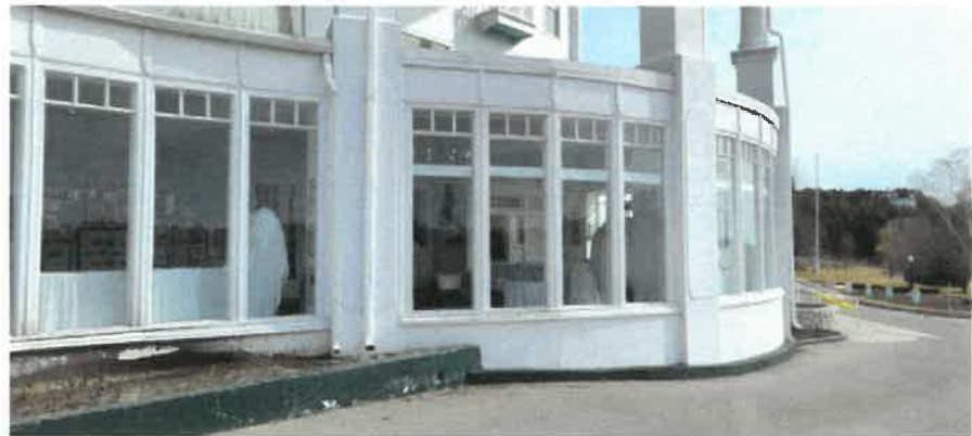
EXISTING EAST LOBBY WINDOWS
