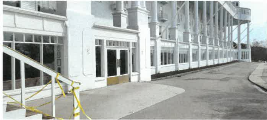
EXISTING EAST LOBBY FACADE
