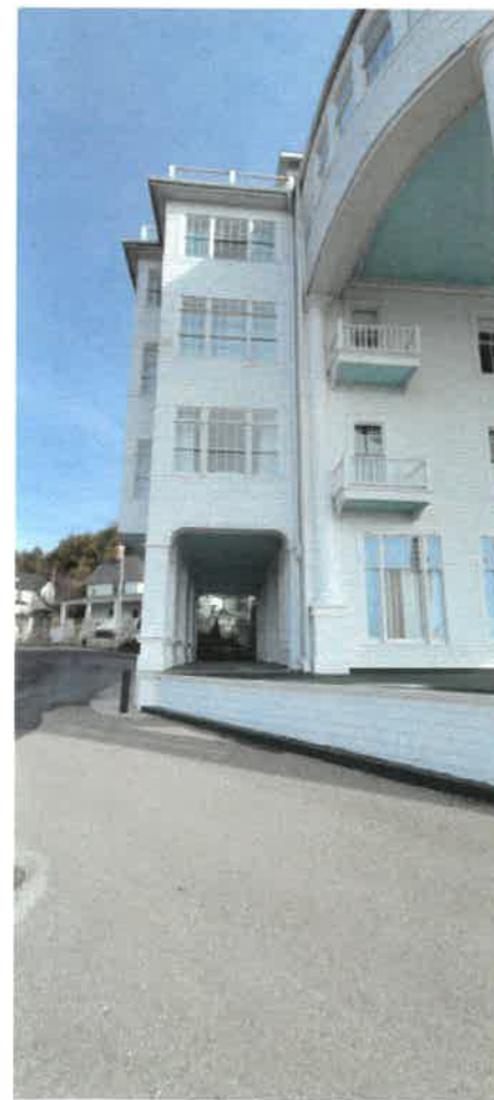
EXISTING VIEW OF WEST END
