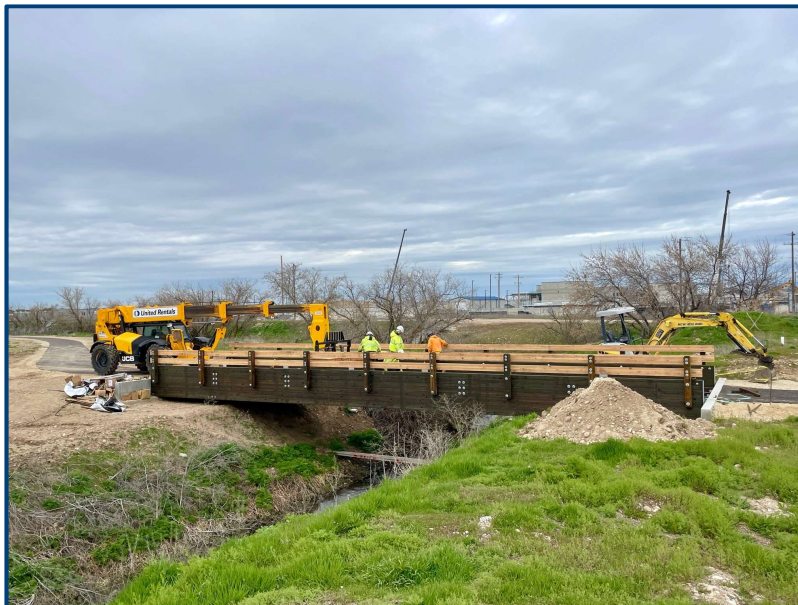
Pedestrian Bridge over Ninemile Creek
