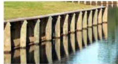
structural bulkhead
