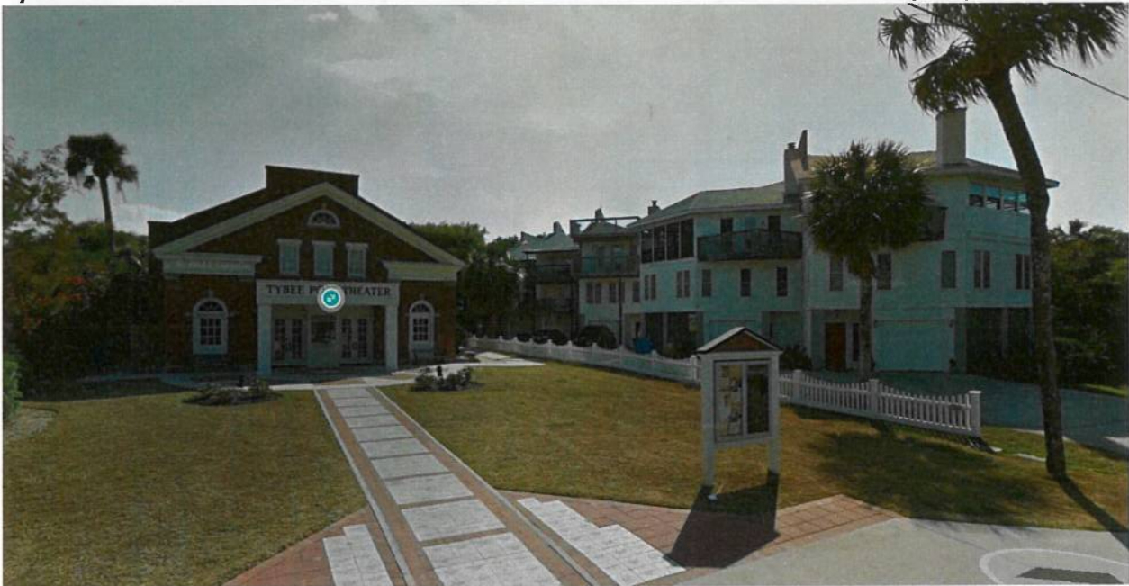
Tybee Post Theatre and 6-unit condominium across Van Horne from the Property:
