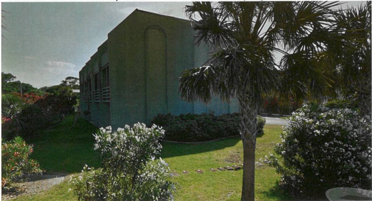
10-Unit Condominium directly across Van Horne from the Property:
