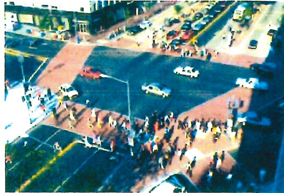
Pedestrian friendly intersections are built at a scale to keep traffic in motion. Overly wide intersections complicate safety, access and pedestrian issues. The above intersection at Connecticut and "K" Streets in Washington, D.C. is an excellent example of a top performing intersection that is not overly wide and accomodates pedestrians. Clearwater, Florida collapsed three nonsignalized and three signalized intersections into one roundabout intersection (below). The alteration allows another 20,000 vehicles to move (40,000 to 60,000), plus it also accomodates 6-8,000 pedestrians on special weekend days at the beach.
