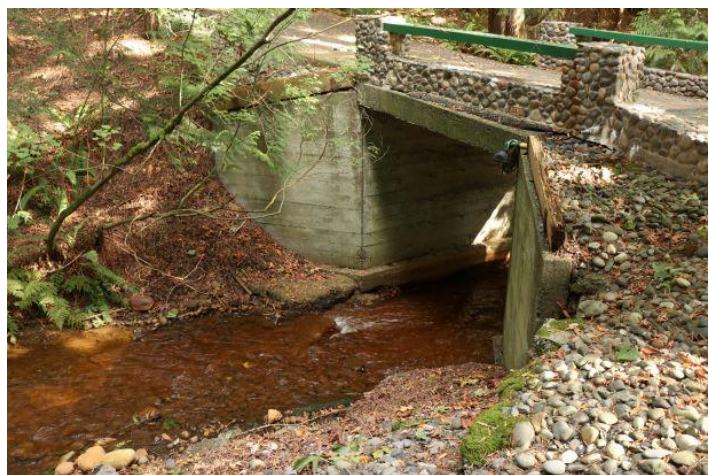
Box culvert bridge on the existing driveway over Pepin
