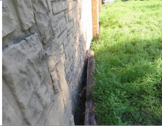
Figure 26 - Wood wall adjacent to panel 39 from yard of 4133 Stinwick Lane.
