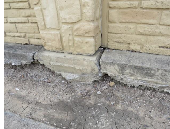
Figure 13 - Typical condition of column foundation and mow strip interface along wall.
