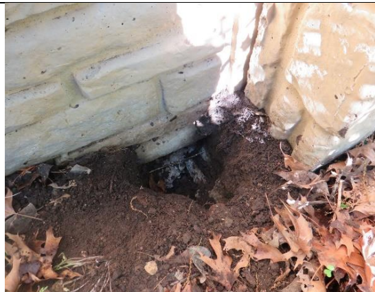
Figure 28 - Column foundation visible at base of column near panel 42.
