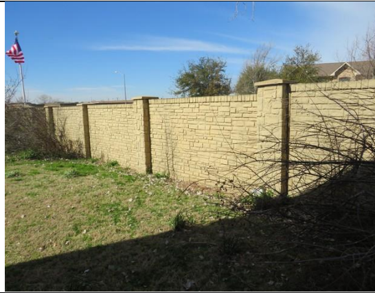
Figure 8 - Interior view of screen wall at backyard of 2959 Chanute Drive.
