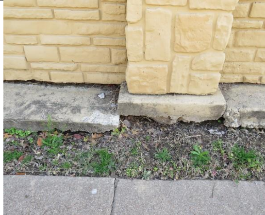
Figure 14 - Typical condition of column foundation and mow strip interface along wall.
