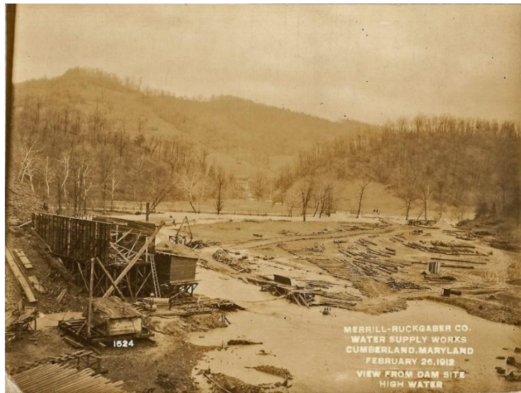
Figure 1: Lake Gordon Dam Construction 1912
