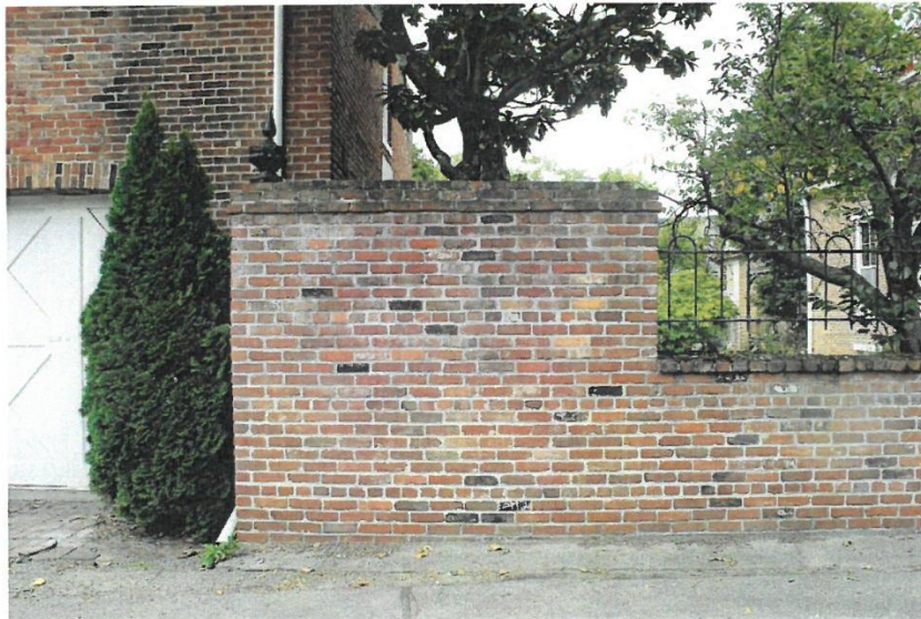
South end cap wall, facing west
