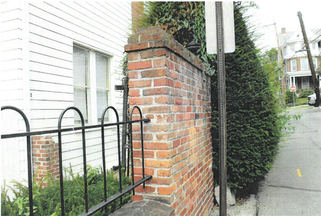
Northern endcap wall, facing north.
