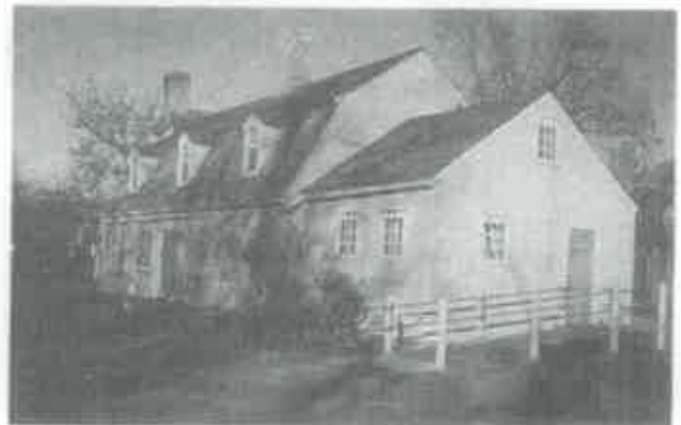
Figure 7. This ramp is convenient for visitors with disabilities and preserves the building's historic character. The design is also compatible in scale with the building. Photo: William Smith.
