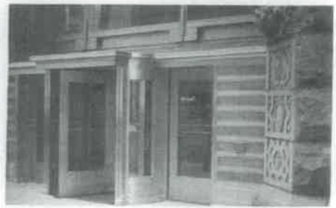
Figure 16. During the rehabilitation of the Rookery in Chicago, the original entrance was modified to create an accessible entrance. Two revolving doors were replaced with a new one flanked by new doors, one of which is operated with a push-plate door opener. Photo: Thomas Jester.
