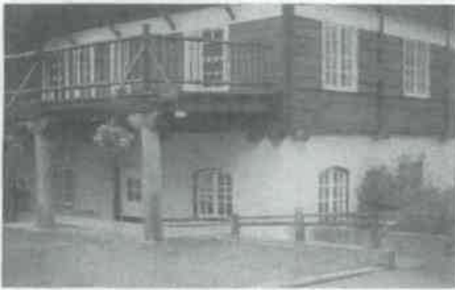
Figure 8. A new below-grade ramp provides access to Lake MacDonahí Lodge in Glacier National Park. Photo: Thomas Jester
