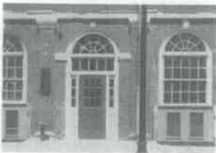
Figure 15. A new entrance to the elevator lobby replaces a window at Faneuil Hall in Boston, Massachusetts. The new entrance is appropriately differentiated from the historic design. Photo: Paul Holtz.
