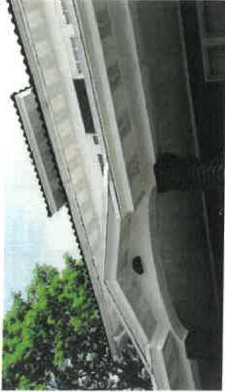
Guideline 34: Undesirable treatment of historic porch features. Though the porch retains the overall massing and proportions, all of the porch details have been sheathed in synthetic siding.
