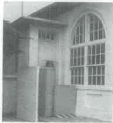
Figure 13. Platform lifts like the one used on this building require minimal space and can be removed without damaging historic materials. Shielded with lattice work, this lift is also protected by the roof eaves. Approach path should be stable, firm, and slip resistant. Photo: Sharon Park
