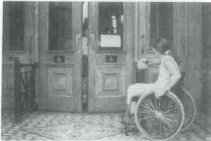
Figure 5. A universal access symbol clearly marks the Arts and Industries Building in Washington, D.C., and a push plate (right) engages the automatic door opener. Photo: Thomas Jester.
