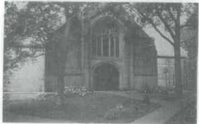
Figure 6. Entrances can be regraded to make a building accessible as long as no significant landscape features will be destroyed and as long as the building's historic character is preserved. The Houghton Chapel (a) in Wellesley, Massachusetts, was made accessible by regrading over the historic steps (b). Photos: Carol R. Johnson & Associates.
