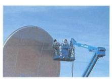
Soda blasting a radio dish at Hat Creek Radio Observatory
