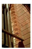
Brick molding next to the window has been severely abraded by sandblasting to remove paint. Photo: NPS files.
