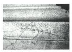
Very high-pressure water has scarred this granite. Photo: NPS files.
