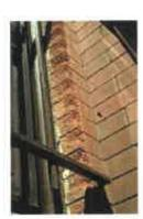
Brick molding next to the window has been severely abraded by sandblasting to remove paint. Photo: NPS files.
