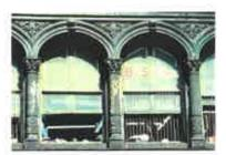
Cast iron may be abrasively cleaned, but must be painted immediately to prevent rust. Photo: NPS files.
