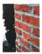
Abrasive cleaning can cause permanent damage to historic fabric, such as this brick wall. Photo: NP5 files.
