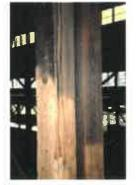
Industrial Interiors that are not finally milled may be abrasively cleaned, in some instances, Photo: NPS files,
