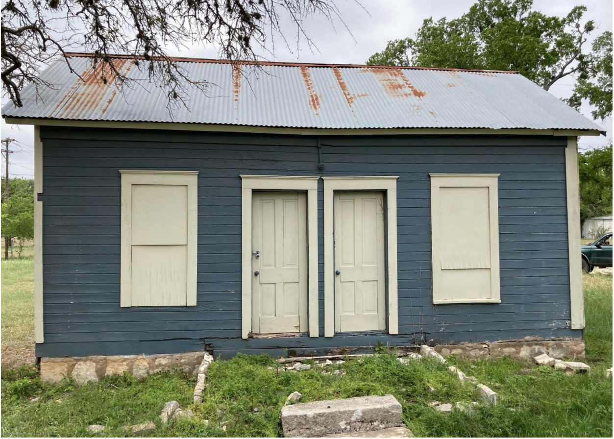
215 Fitzhugh Road / Front Facade
