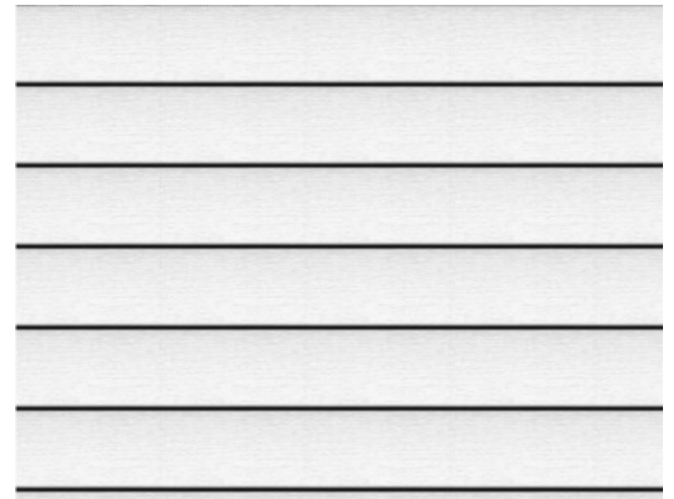
Painted Horizontal Lap Siding on new Kitchen addition (painted White to match)
