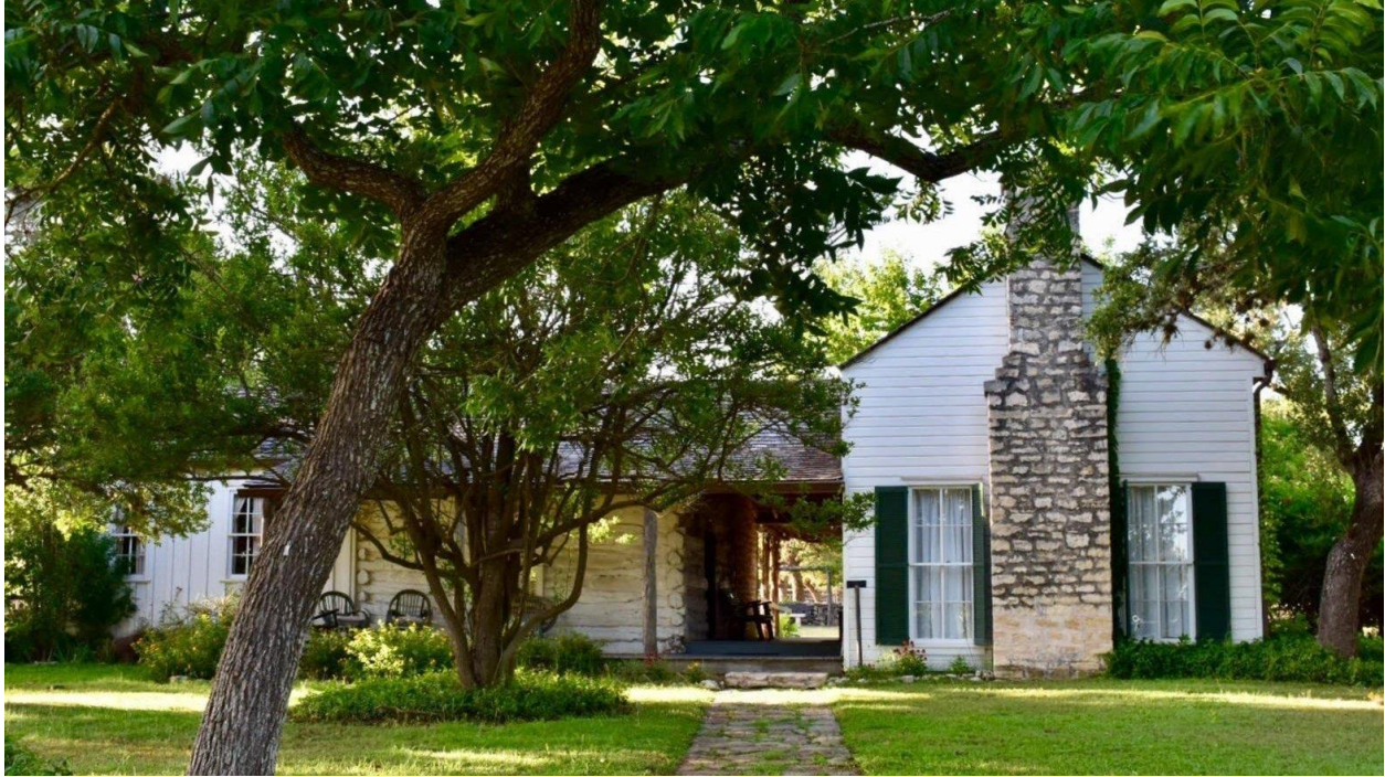
Existing conditions: front porch view of Pound House. Image sourced from Pound House Museum.
