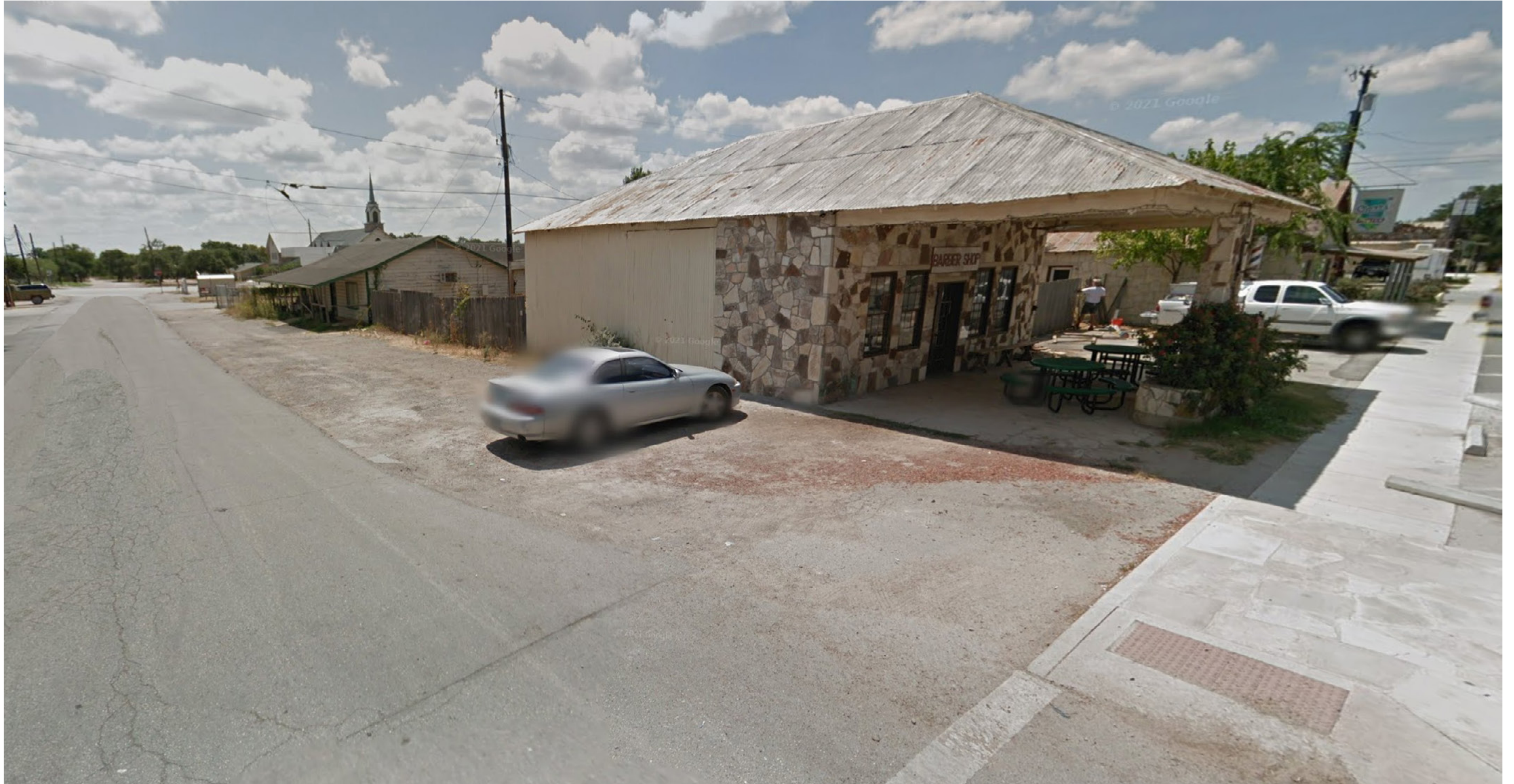
Existing structure from corner of Mercer Street and San Marcos Street
