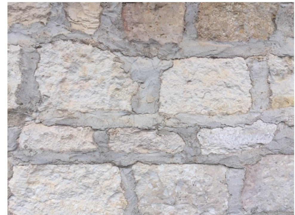
Native Limestone Veneer at New Porches, HVAC Screen Wall and Dumpster Wall to be similar to Short Mama's house and Garage out-building
