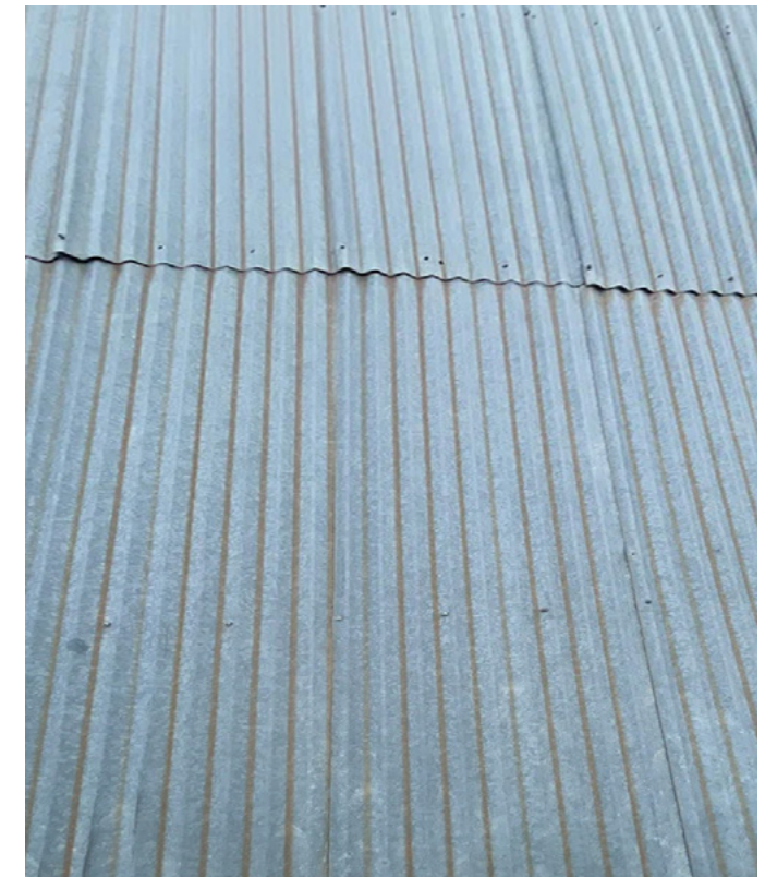
Reclaimed metal panel from existing wood shed
