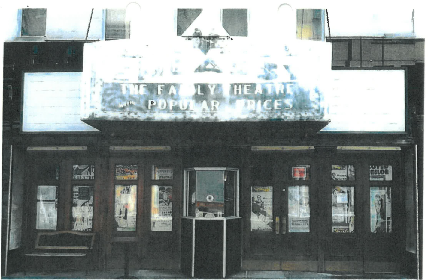
Figure 1 – Front of Embassy Theatre building, February 2015
