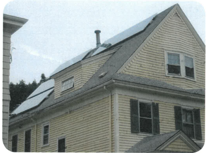
These solar panels low profile and location make them unobtrusive even though they are visible from the public right of way. Photo by Paul Trudeau
