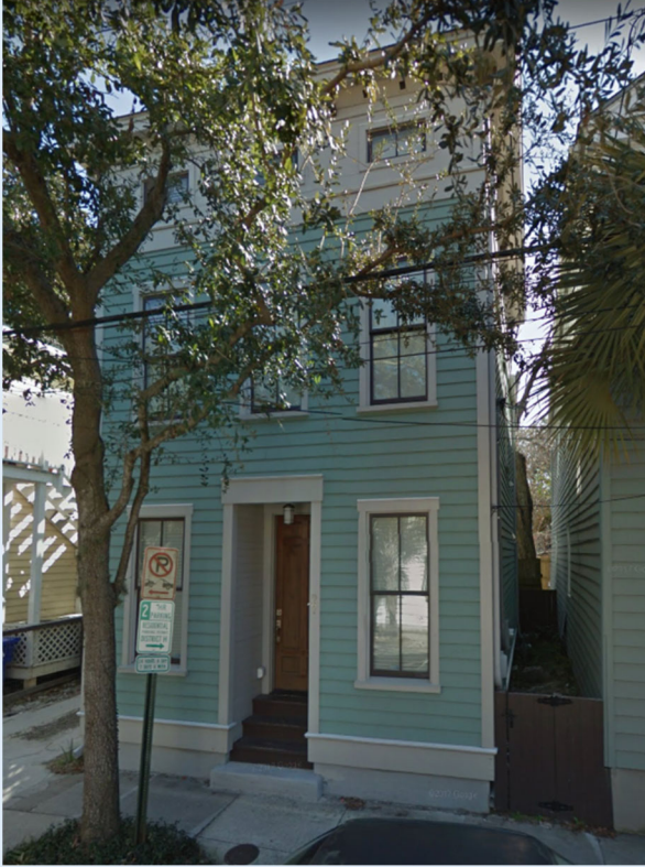
Lowered siding and windows on new structures only
