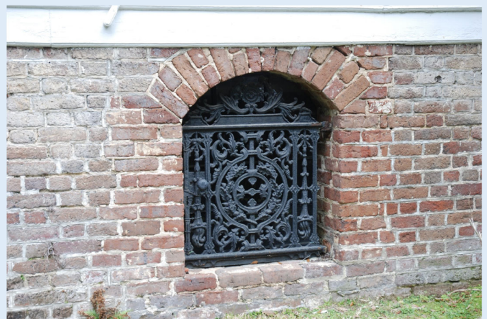
Decorative ironwork at venting
