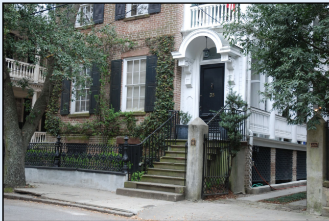
Coping Walls & Fencing
