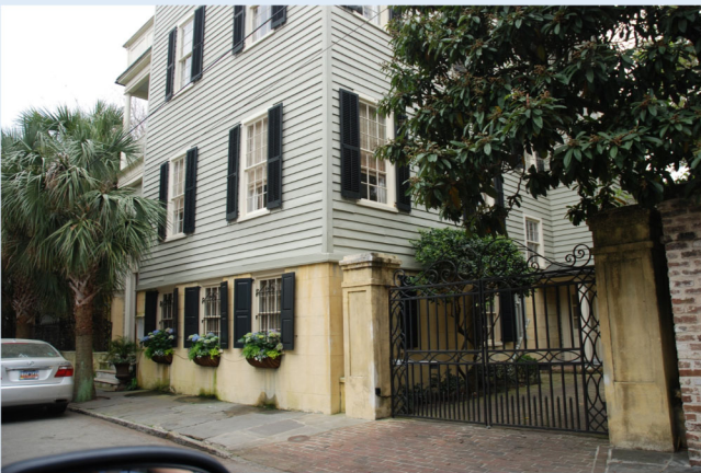
Fenestration in foundation
