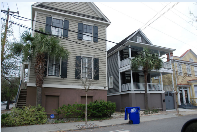
Solid foundation at front
