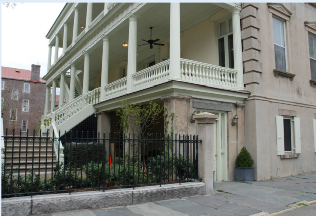
Extension of column line to pier foundation
