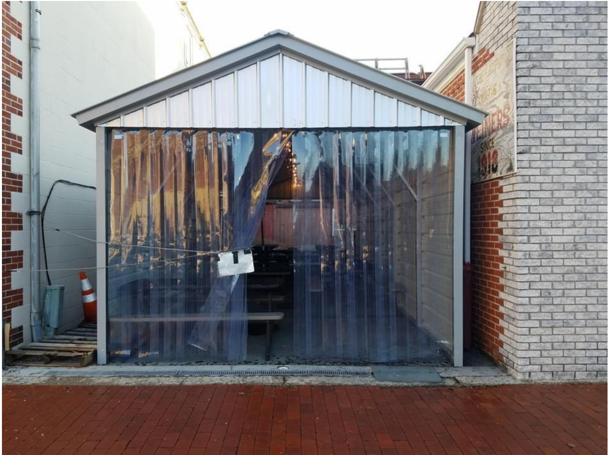
After Carport Installation
