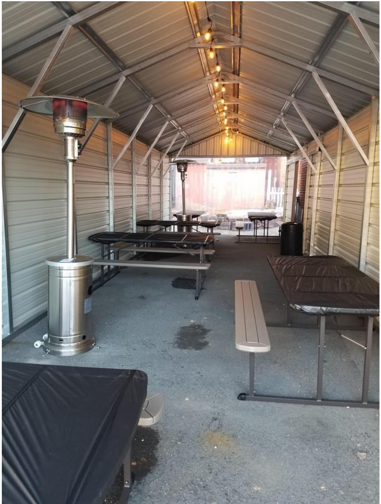
After Carport Installation
