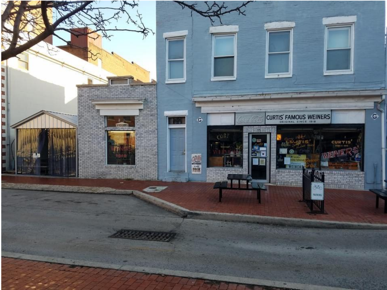
After Carport Installation
