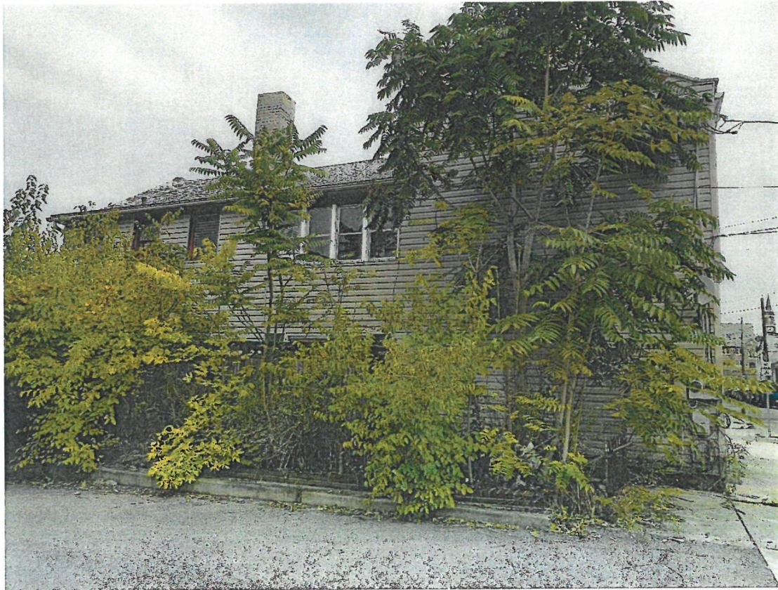
Photo 4 – View of West side of dwelling. Shrubbery has overgrown and should be removed.
