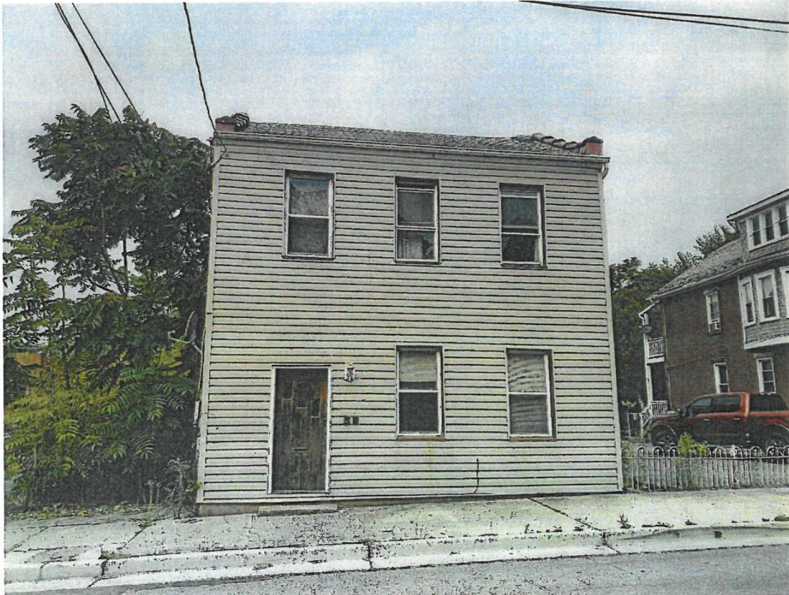
Photo 1- Front or South side of dwelling facing Polk Street.
