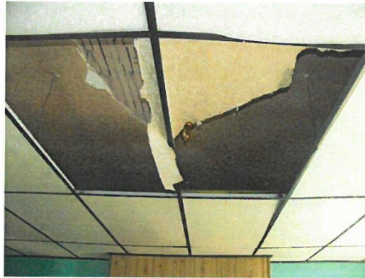
Ceiling in Living Room
