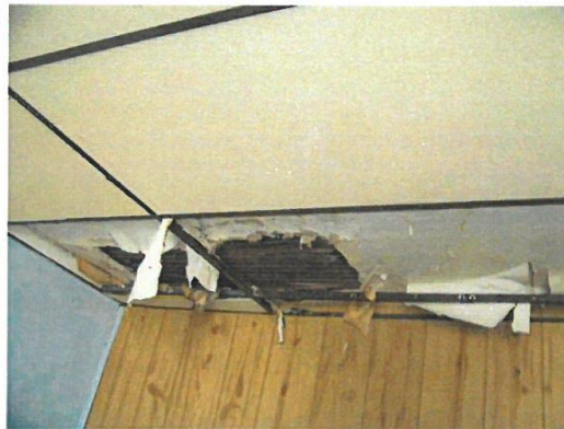
Ceiling in Living Room
