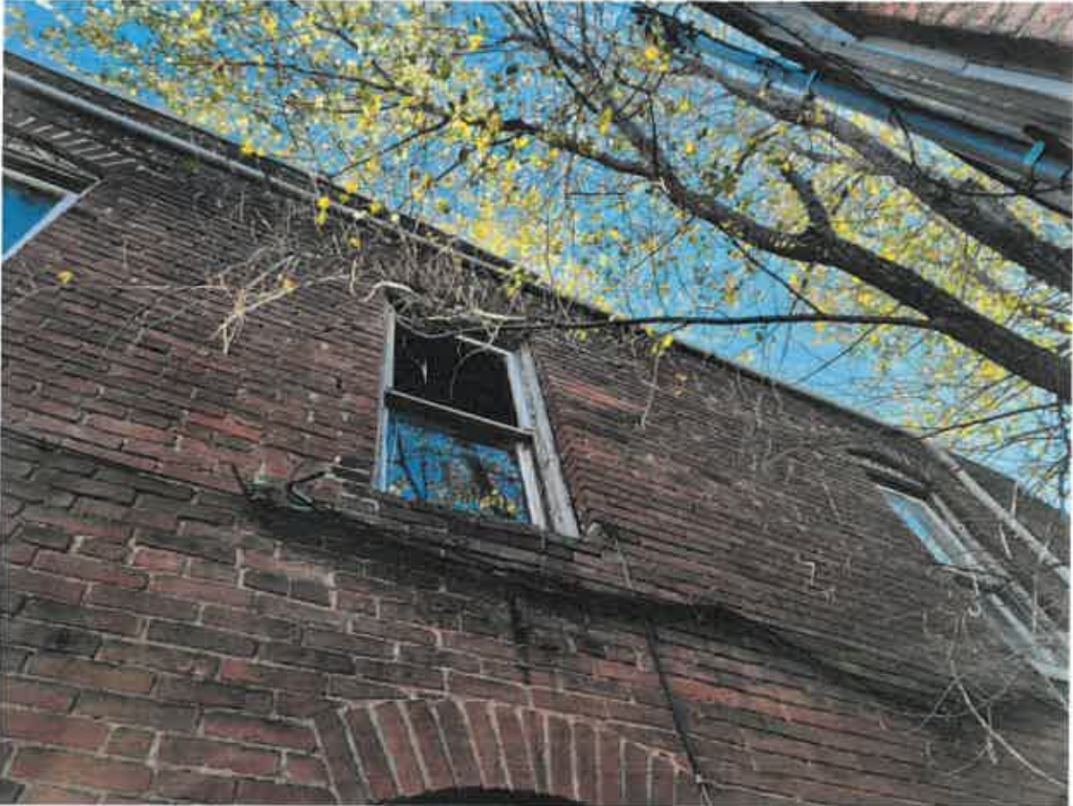
Photo 2. North side of building.
