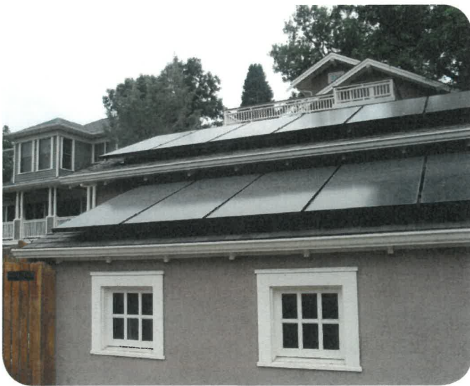
Solar panels placed on an accessory structure not visible from the public right of way should still follow the slope of the roof and have a low profile. Photo courtesy of Dan Corson
