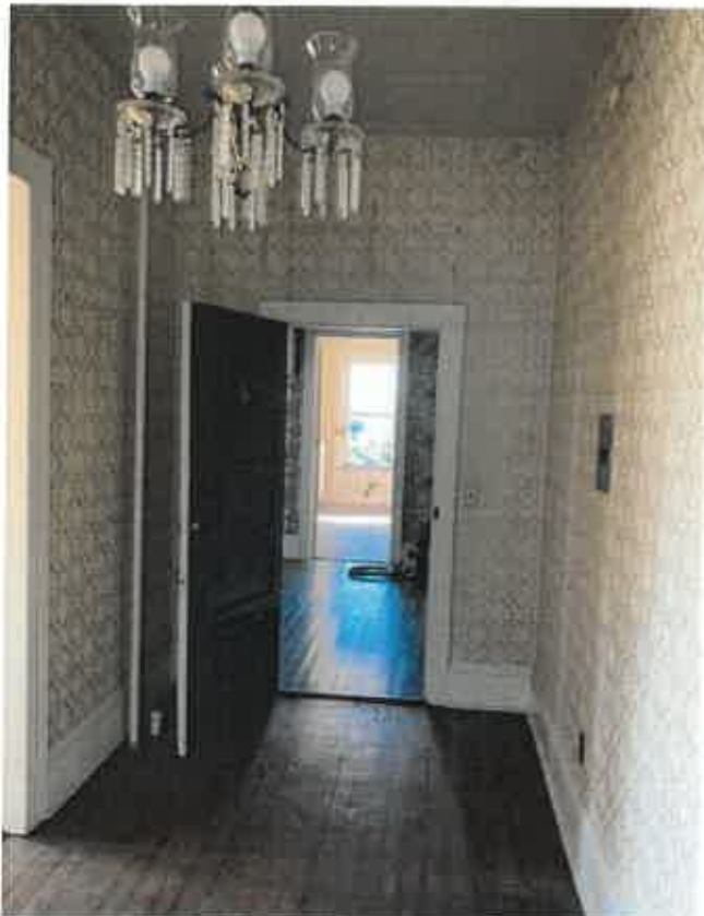
Panel doors into Apartment 3 (near door) and Apartment 4 (far door) need to have fire retardant backing
