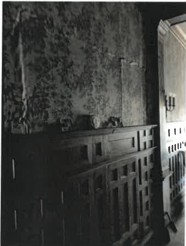
Main floor hallway plaster repair (this is palimpsest of the pocket door entrance to the original dining room) and wall-papering to be done.
