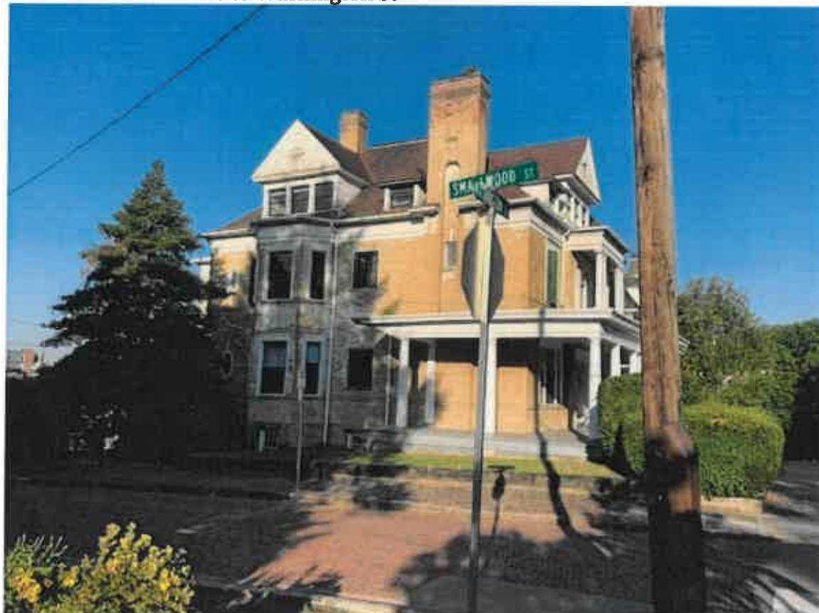
Smallwood Street side to Washington St
