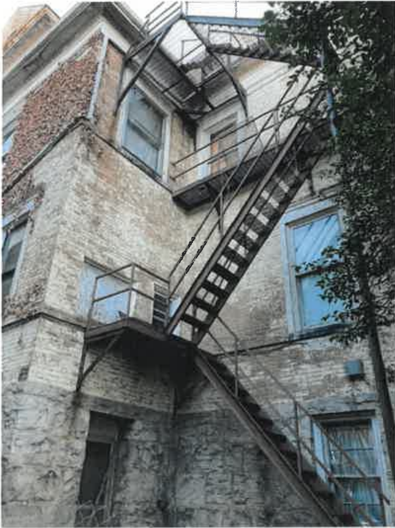
Side toward next door house, 206 Washington St.
