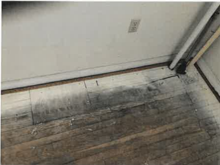
Apartment 1 carpet stretchers removed and oak floor sanded and finished.
