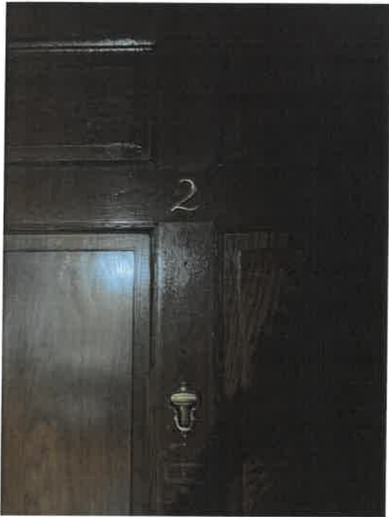
Panel doors into Apartment 3 (near door) and Apartment 4 (far door) need to have fire retardant backing
