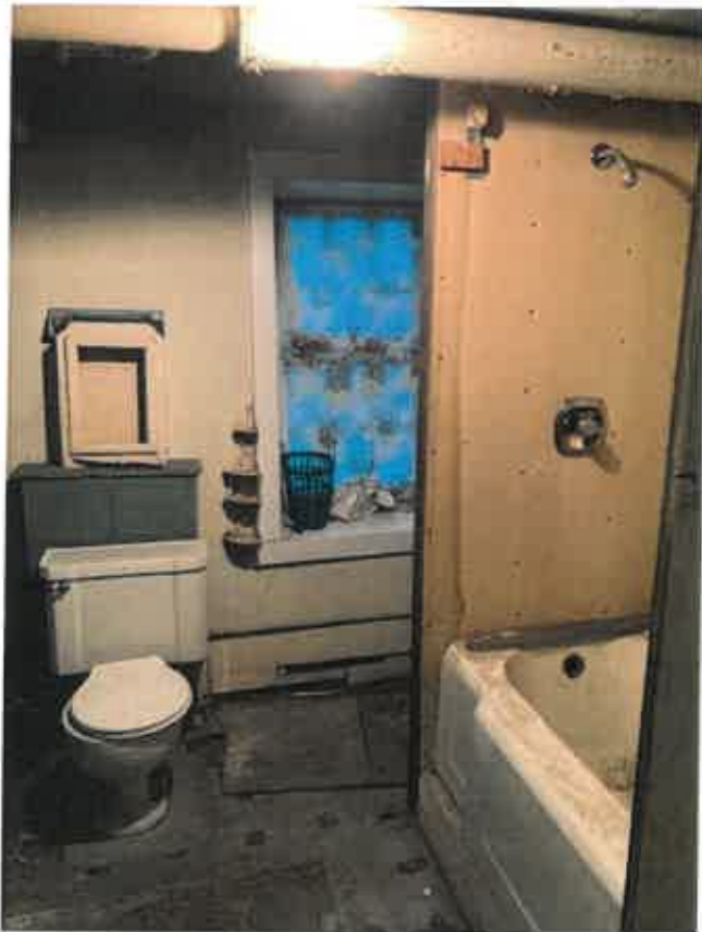
Apartment 6. Tile floor, new water-efficient toilet, new faucets, tile tub-surround.
