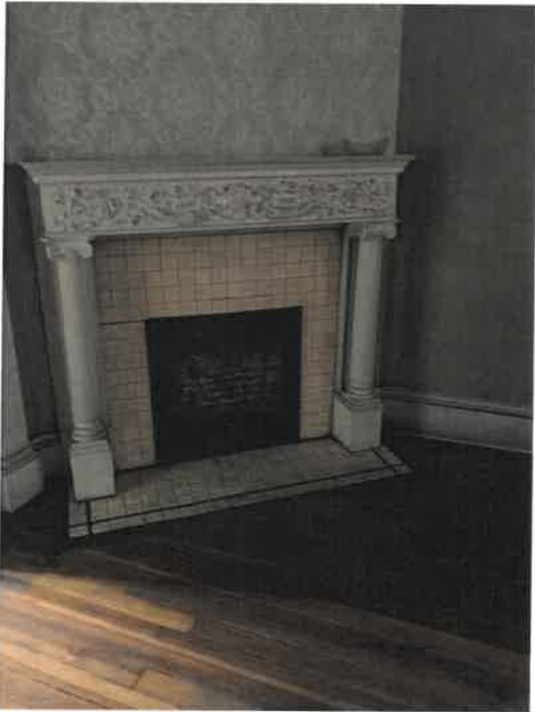
Apartment 3 fireplaces and mantles. Paint touch up—no tile work needed
