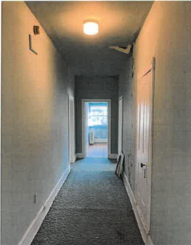
3 rd floor corridor carpeting to be removed. Fir floor to be sanded and finished.
