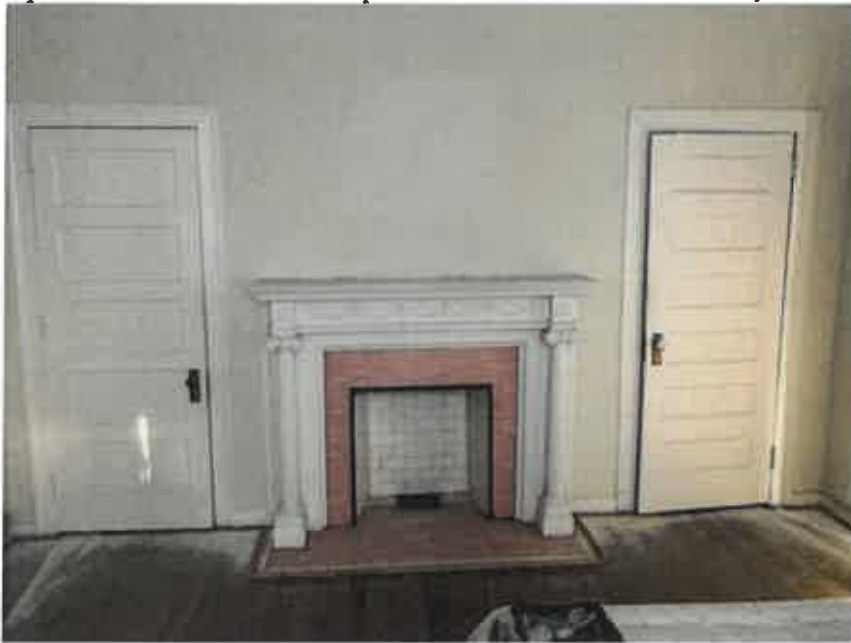
Apartment 1 living room carpet stretchers to be removed, oak floor sanded and refinished.
