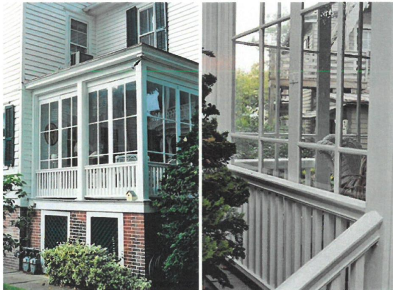
Figure 12. This old porch enclosure, located on the back side of a house, has acquired significance over time and is remarkable both in the appropriateness of its detailing for use by others today, as well as its high degree of maintenance. The enclosure is set behind the columns; the balustrade has been retained; and the light divisions and the size of the glass panes echo that of the windows above. Within each bay there are two well-crafted, inward swinging doors, providing for greater seasonal use of the porch. Photos: Charles Fisher.
