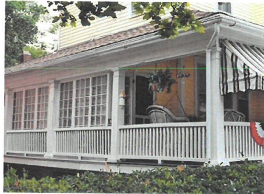
Figure 15. A traditional technique of porch enclosures still used today involves the insertion in each column bay of one or more glass enclosures set in wood frames. This enclosure is properly set back an entire porch bay from the front of the house and utilizes traditional light divisions and wood frames. The balustrade, added here for illustration purposes, shows the importance of retaining this linear feature within the enclosed bays. Photo: Charles Fisher.
