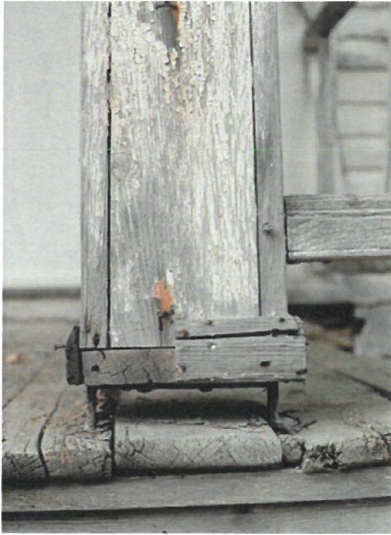
Figure 6. A traditional way to extend the life of porch posts was to place posts on metal feet, thereby providing a separation between the wood post and wood deck. This helped to prevent the wood post from rotting at the base. Early post feet were simple iron bars bent into a stirrup shape. By the late nineteenth century manufactured cast-iron feet were common, consisting of a pair of disks separated by a short pipe. Post feet are still available today. Courtesy of Old-House Journal/Brian McNeil.
