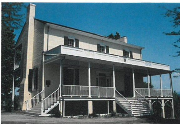
Figure 2. Porches not only help define the architectural character of a building but also serve as living areas. They can be designed to take advantage of surrounding views. Cedar Grove, the home of the nineteenth-century landscape painter Thomas Cole, has an L-shaped veranda on the front and a two-story porch on the rear, providing an enviable view of the Catskill Mountains. Photo: Marilyn Kaplan.
