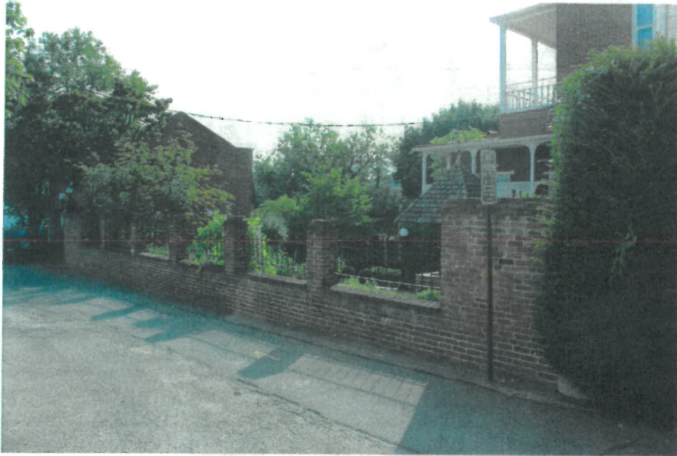
Overview of the eastern perimeter wall adjacent to Spruce Alley showing the low wall topped with metal railing and brick piers, facing southwest.
