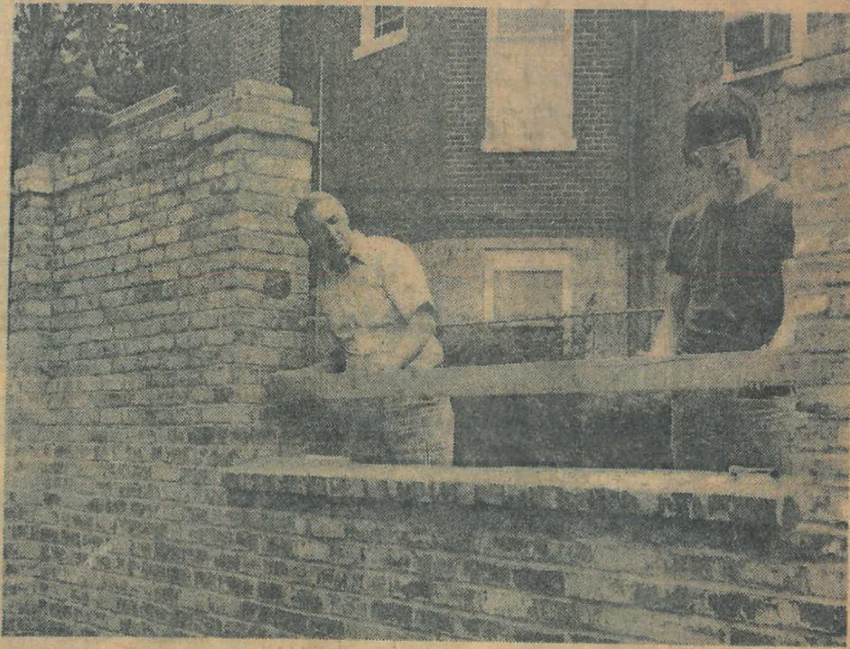
HISTORY HOUSE WALL COMPLETED — Kyle Diehl, left, masonry instructor at Allegheny Vocational-Technical Center, and Mark Edwards, a Vo-Tech student, check the proper spanning of a Bicentennial brick wall project at the Allegheny County Historical Society headquarters, 218 Washington Street. The wall is 200 feet long and from five to eight feet high. Bricks were obtained from the old Cumberland Brewery and urban renewal projects. Other Vo-Tech students assisted and the Vo-Tech welding shop, Vincent King, instructor, fabricated metal fence sections to be placed between brick posts on Spruce alley.
