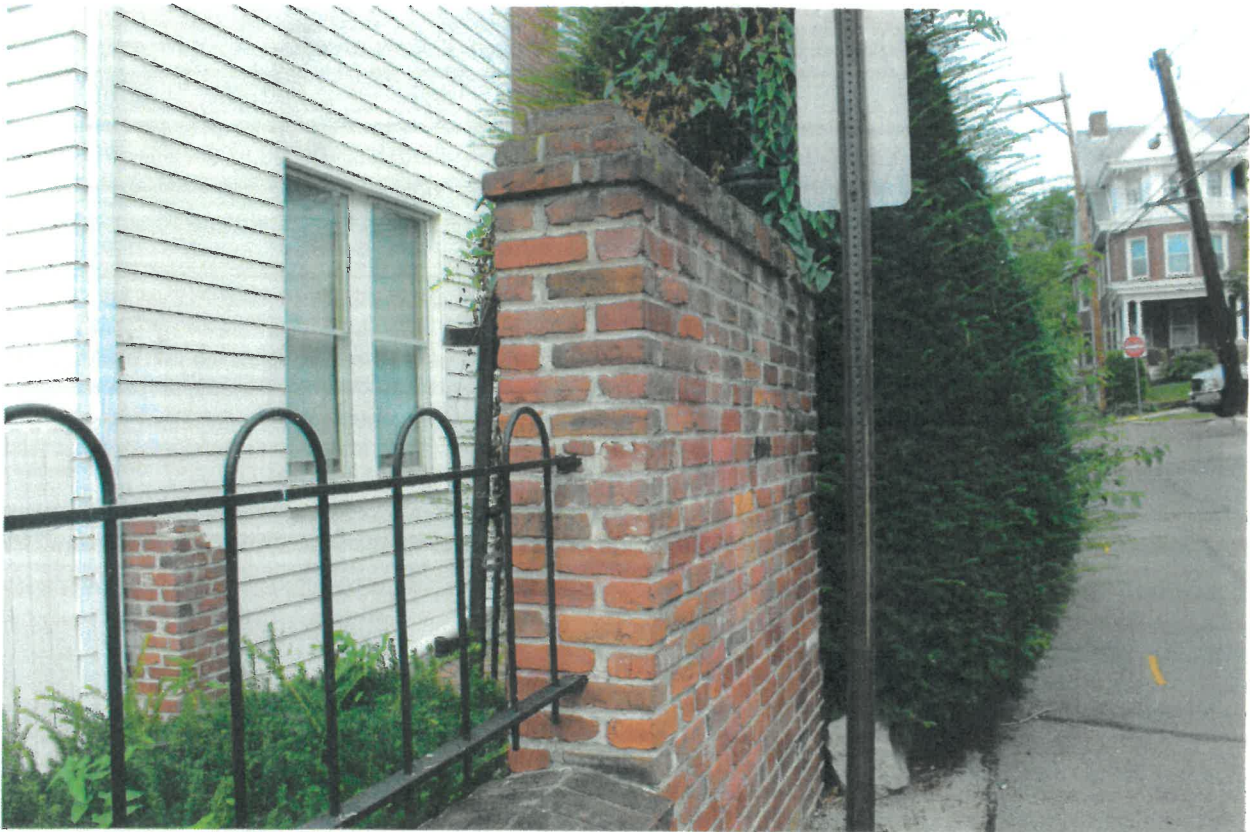
Northern endcap wall, facing north.
