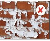
Non-historic paint coatings and water repellent treatments are inappropriate for historic masonry
