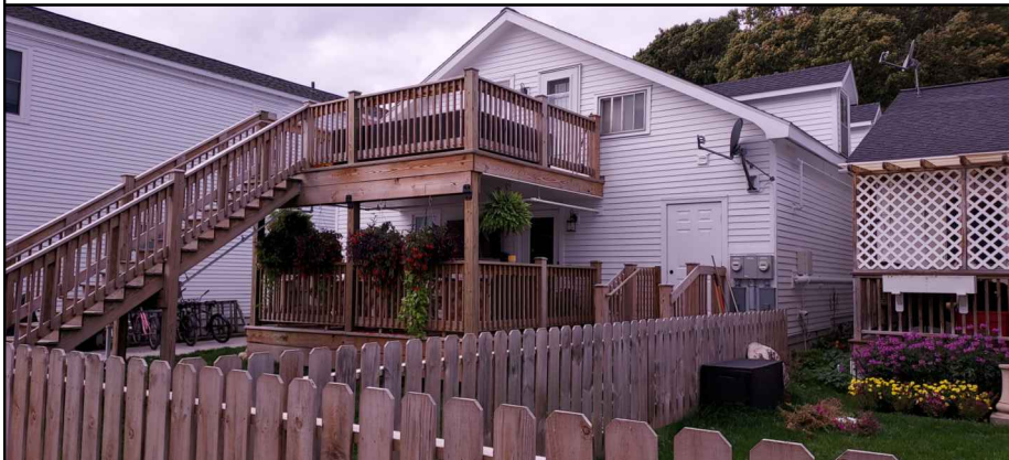
ALLEY VIEW OF GULL
