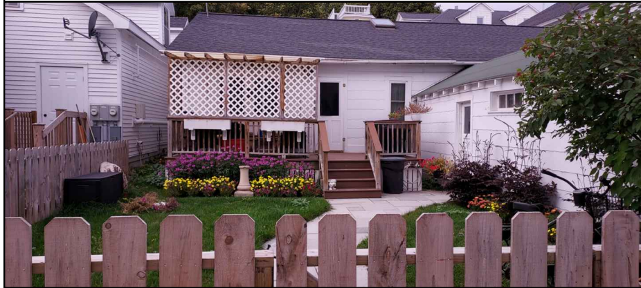
ALLEY VIEW OF EXISTING ROSE UNIT
