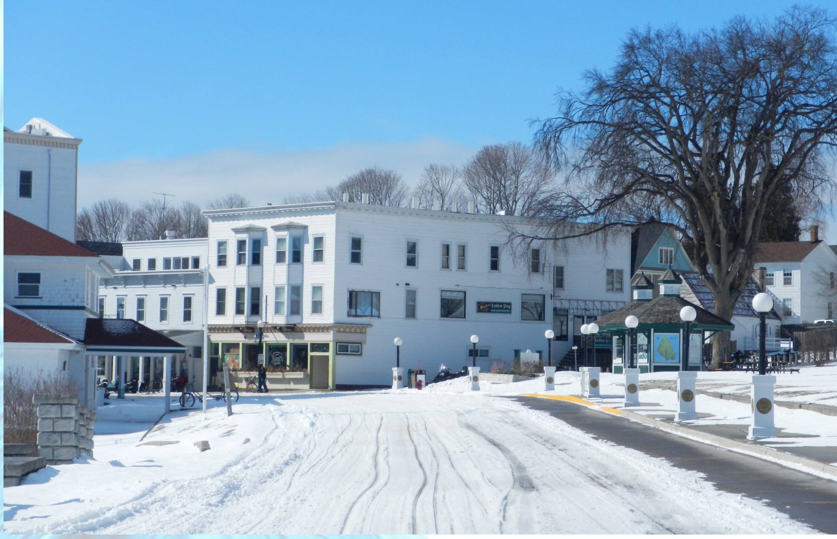
VIEW # 2 (AFTER) Northeast View (Looking Southwest) of building with New Antennas & Equipment
