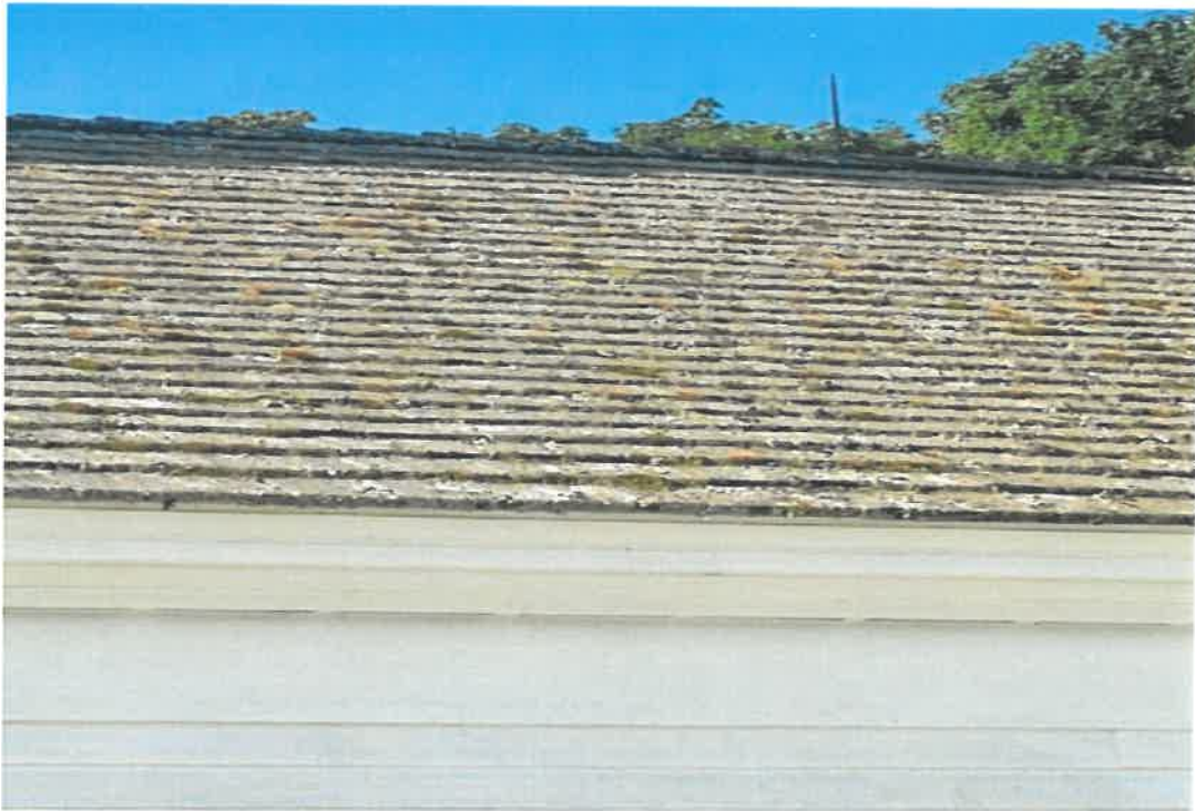
Cedar Shingle Roof
