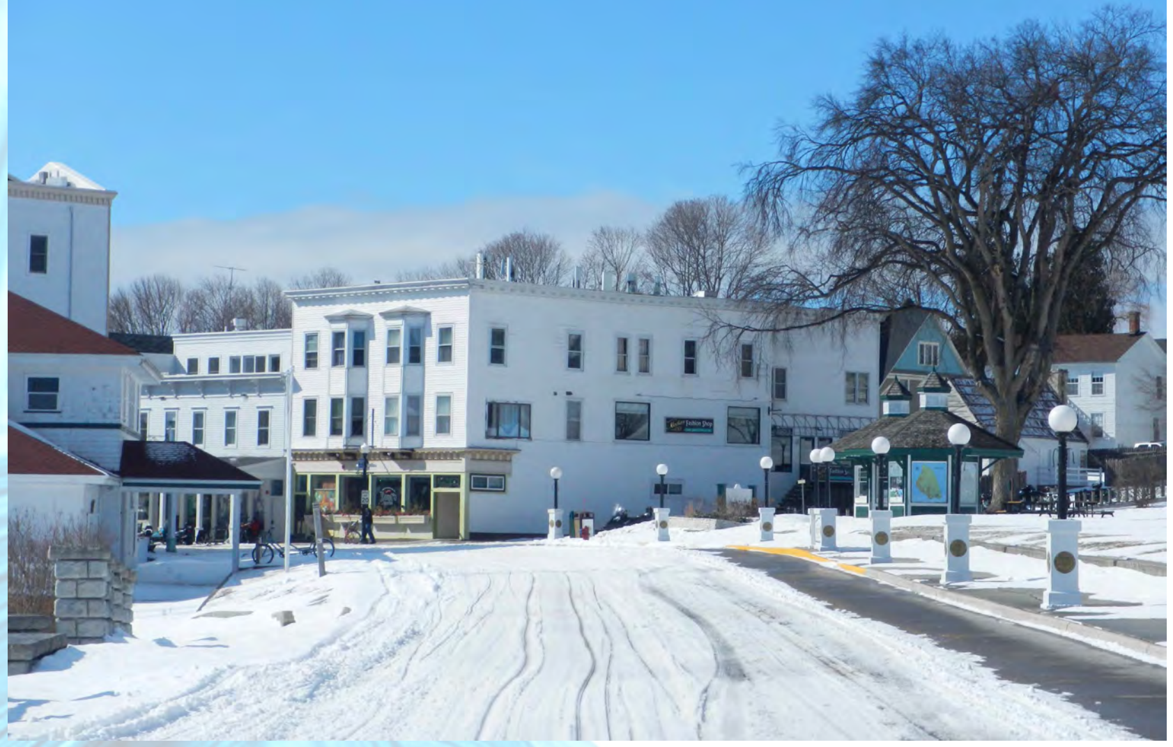
VIEW # 2 (BEFORE) NorthEast View (Looking SouthWest) of building with existing antennas & equipment to be removed
