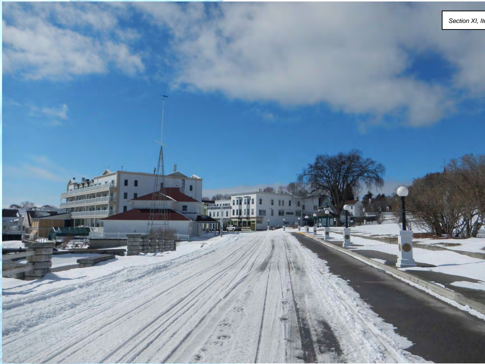
VIEW # 1 (BEFORE) Northeast View (Looking Southwest)
