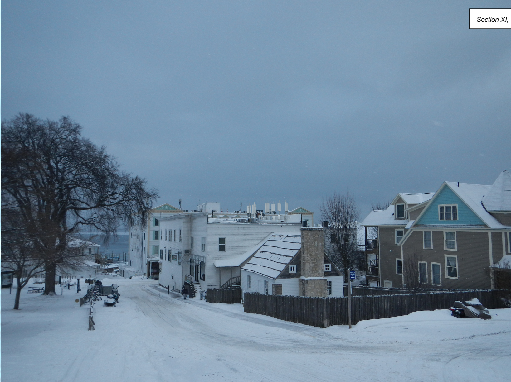
VIEW # 3 (AFTER) Northwest View (Looking Southeast) to building with New Antennas & Equipment
