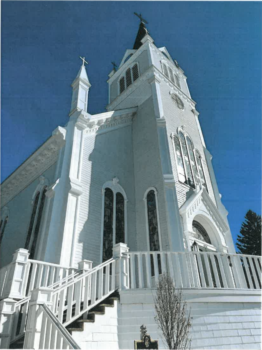
Photo 4. Saint Anne's Church, 6836 Main Street
