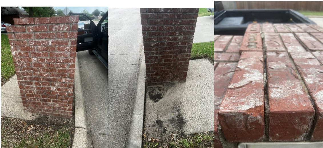
3984-3988 Holly Hill – Top re-done and slab lifted
