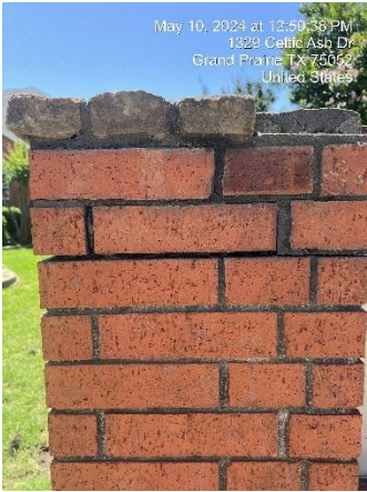
1342-1346 Ashbrook Dr – Top re-done and slab lifted
