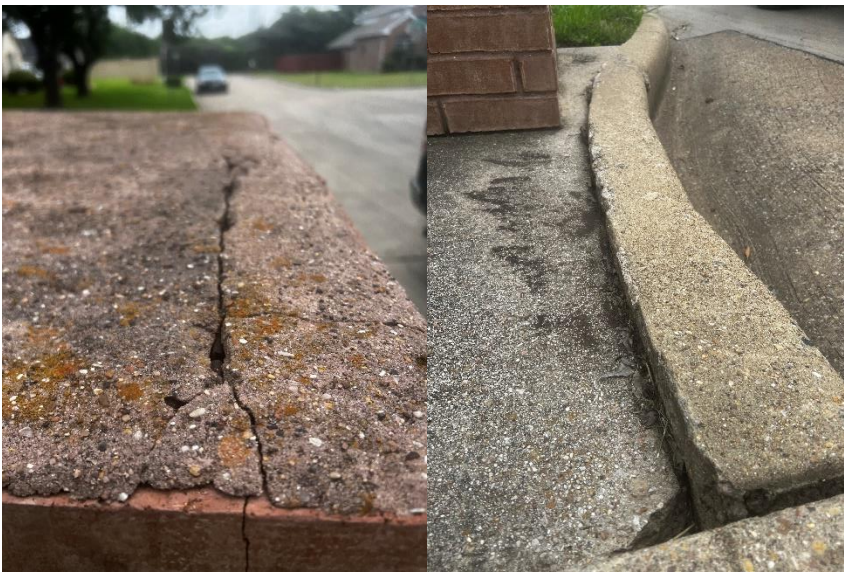
3984-3988 Holly Hill – Top re-done and slab lifted
