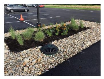
Figure 10: An HPMBS basin installed at a parking lot catch basin. The total footprint of the practice is about the size of one parking space.
