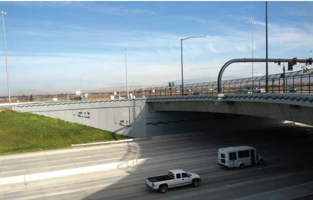
..... Below: Bridge deck of the Ten Mile Interchange over I-84
