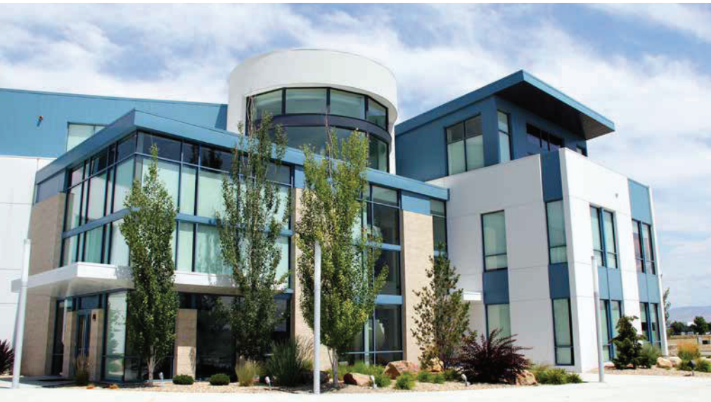
..... Below: The PKG building on Pine Ave
