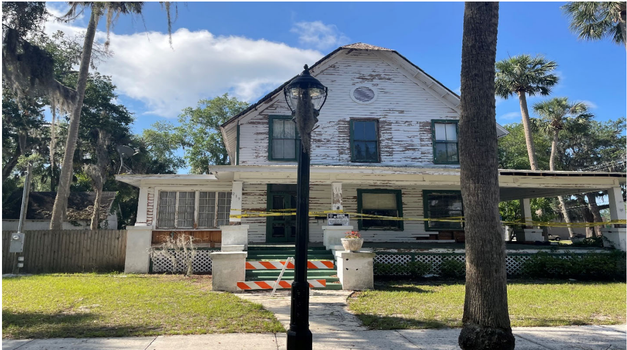
Photo 1: Front of structure
