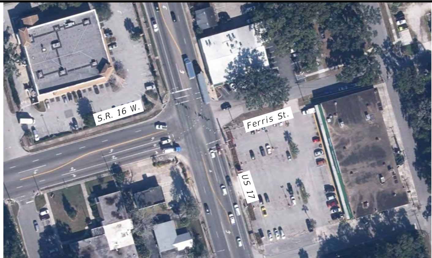
S.R. 16 W. and Ferris Street at US 17
